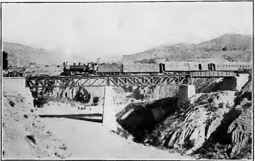
BRIDGE OVER A RECENTLY CONSTRUCTED HIGHWAY CONNECTING LA PAZ AND CHIJINI STATION.
